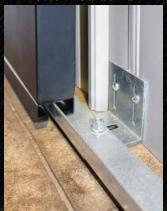
Provides door stability for large sliding doors in windy conditions as well as assisting with door alignment when opening and closing.
